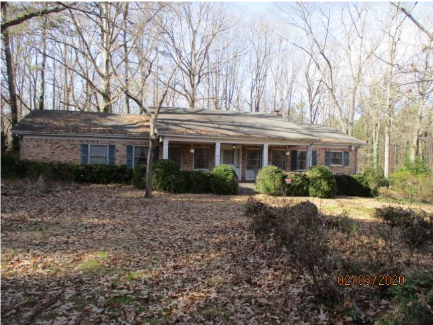
Close-up of Existing Single-Family Residence
