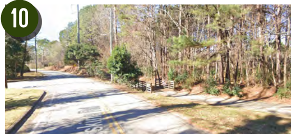
PATH Trail Segment
