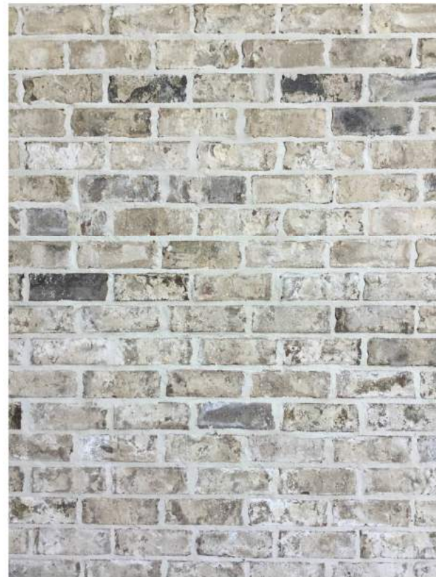
BRICK - MAIN HOUSE BODY CHEROKEE BRICK - BROOKHAVEN GEORGIA CLASSIC MODULAR SIZE - 3 5/8" x 7 5/8" x 2 1/4"
