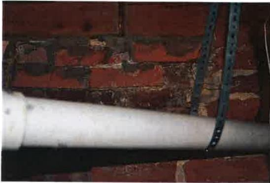
Existing brick cavity stem walls throughout show multiple attempts to point, patch and stabilize settling damage. Attempts as late as 3 years ago are already showing signs of failure.
