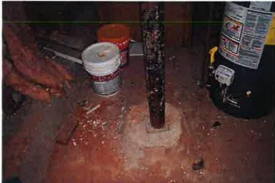
Retrofit steel bracing is supporting over-spanned floor joists, inadequate beams, and a suspended concrete slab. This level is rendered effectively unusable although the bracing employed is still insufficient.
