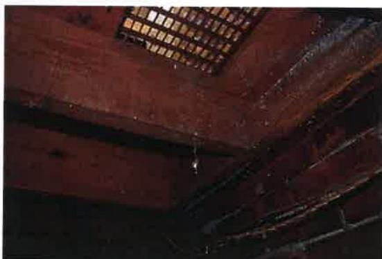
2x8 Floor joists are over spanned 36" average. Sagging entry level floors have been supported via multiple screw jacks in the Crawl/basement. However, 2<sup>nd</sup> floor joists would require removal of all ceilings, electrical and plumbing to facilitate 'sistering' of all joists.
