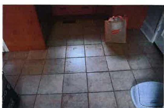
Walls on the upper-level present cracks over doorways, windows, and throughout walls in every room. Baseboard trim illustrates the movement of the floor joists below via gapping. Bathroom floor tiles have separated, unable to withstand the fluctuation of the over spanned floor joists below. Patching measures can be seen throughout that have already separated significantly in 3 years alone.
