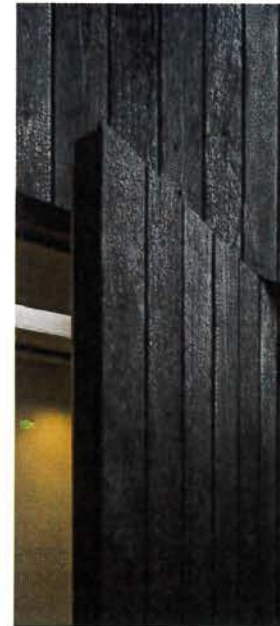
4: ROOF TERRACE WALL
