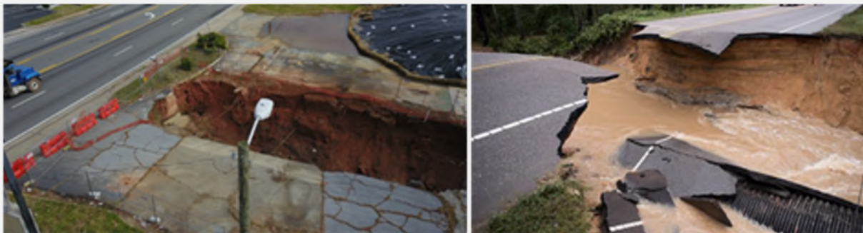
Figure ES-1. Sinkholes and Roadway Washouts Caused by Drainage System Issues
