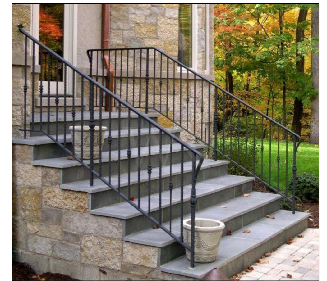
SIMPLE BLACK IRON 36" HIGH GUARDRAIL / HANDRAIL W/ MODEST FLOURISH AT NEELS. NO FLOURISH ON INDIVIDUAL SPINDLES FOR US ALTHOUGH THAT IS SHOWN IN THIS EXAMPLE.
