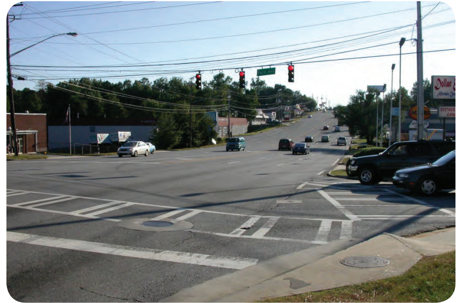
Arterial corridor before (Buford Highway)
