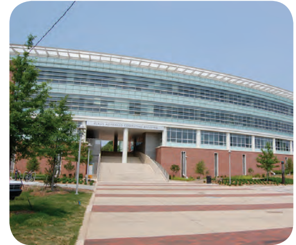
Academic buildings draw a natural set of transit users like students to the TOD
