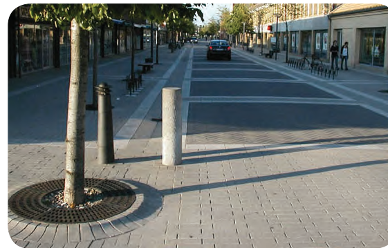
Paving patterns and bollards distinguish between vehicular and pedestrian space.
