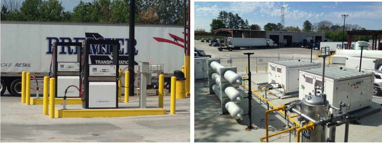
Premier Transportation in Forest Park, GA opened in April 2014.
