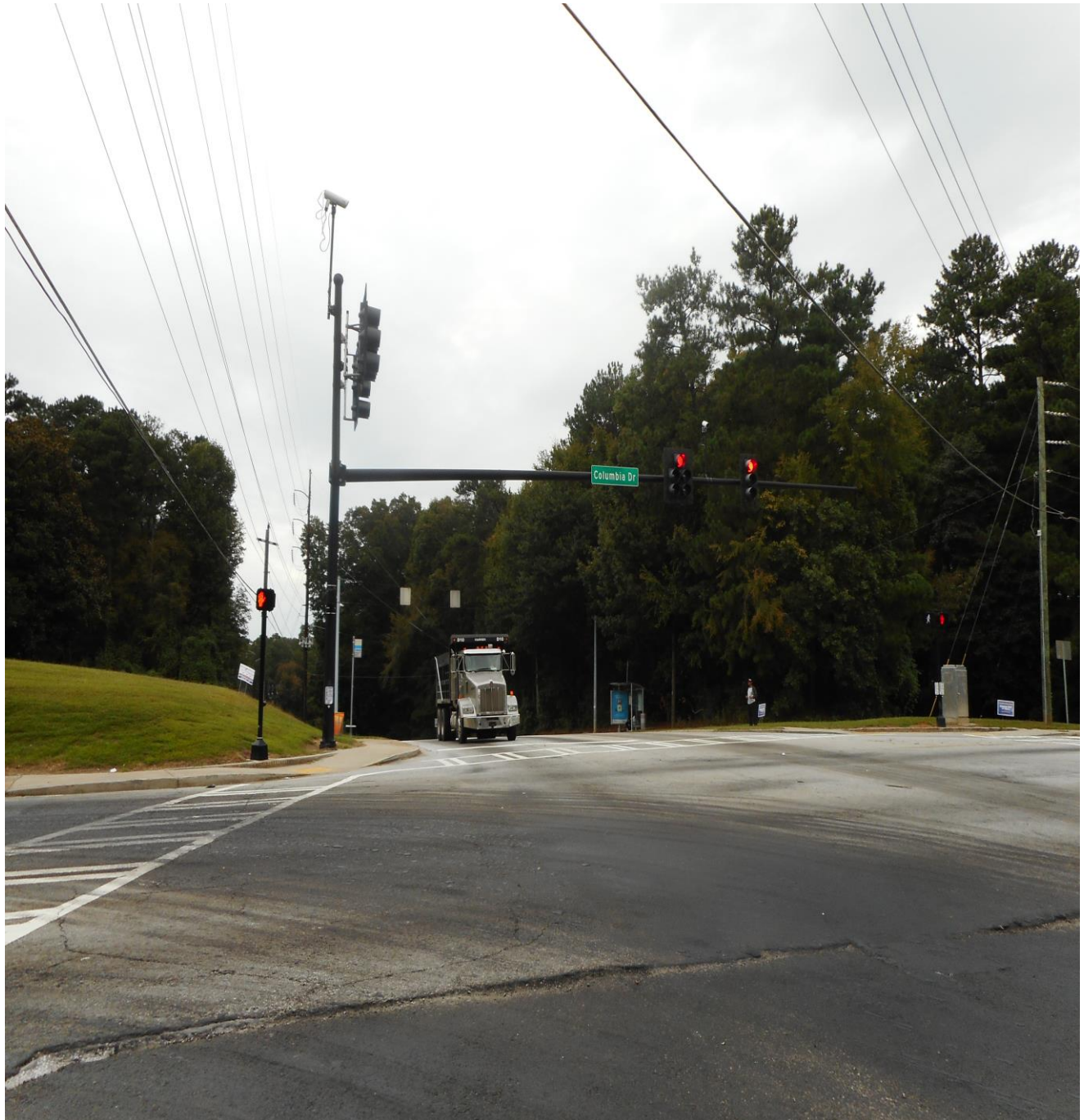
Photograph: View of looking north from the intersection of Columbia Dr. and Rainbow Dr. Taken by Andy B. Anderson September 24, 2020
