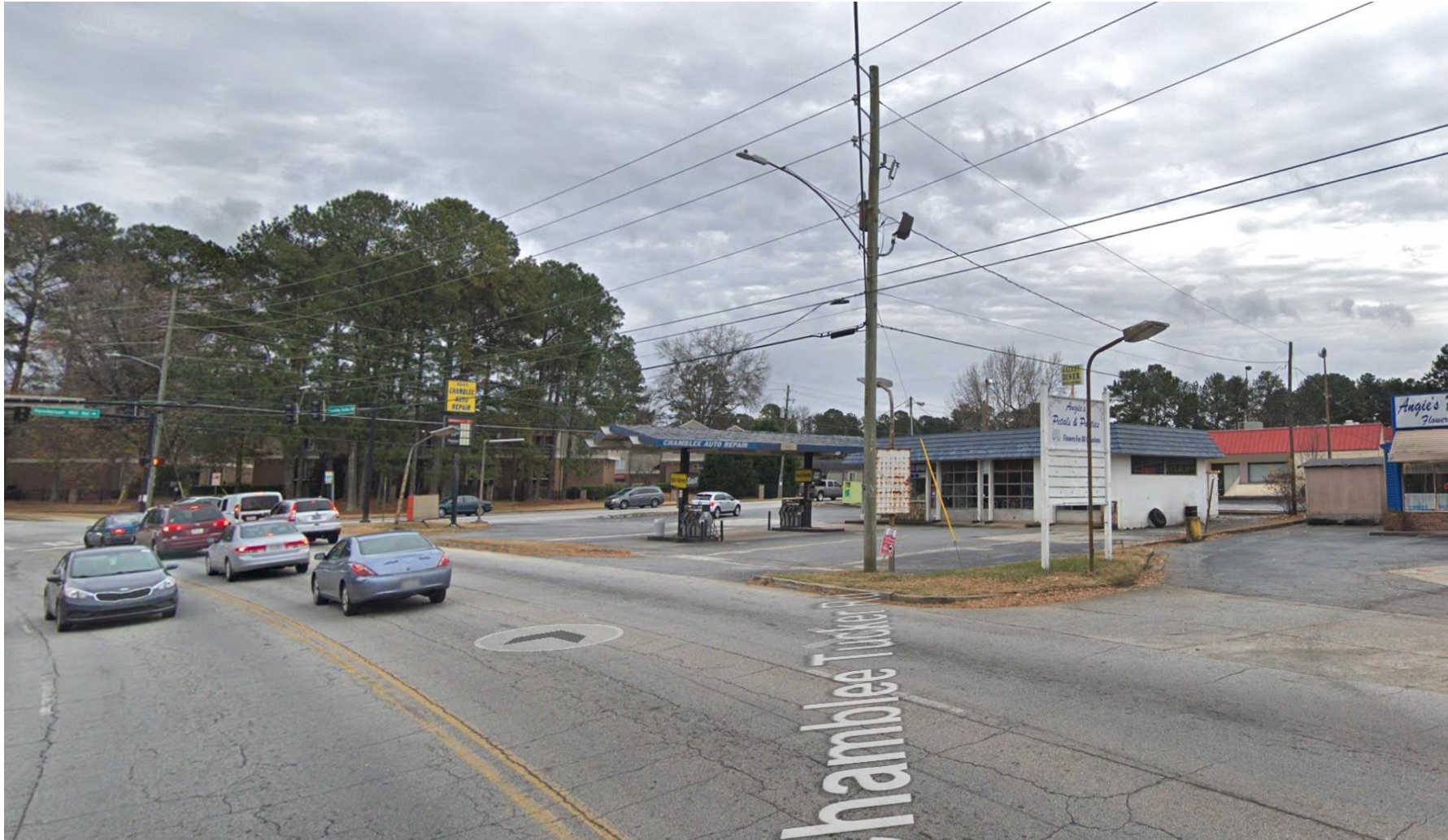
Subject Property, viewed from the northeast
