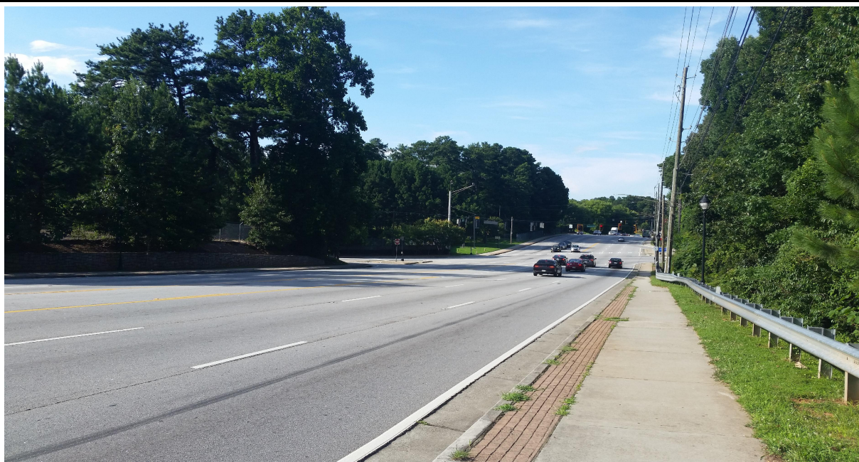
Comments: Site Driveway: Looking north along Memorial Drive (SR 154 / SR 10)
