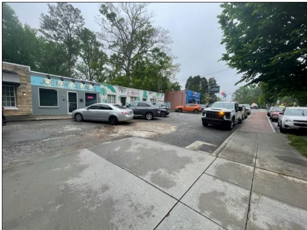
View toward the area to be conveyed by DeKalb County facing northwest.
