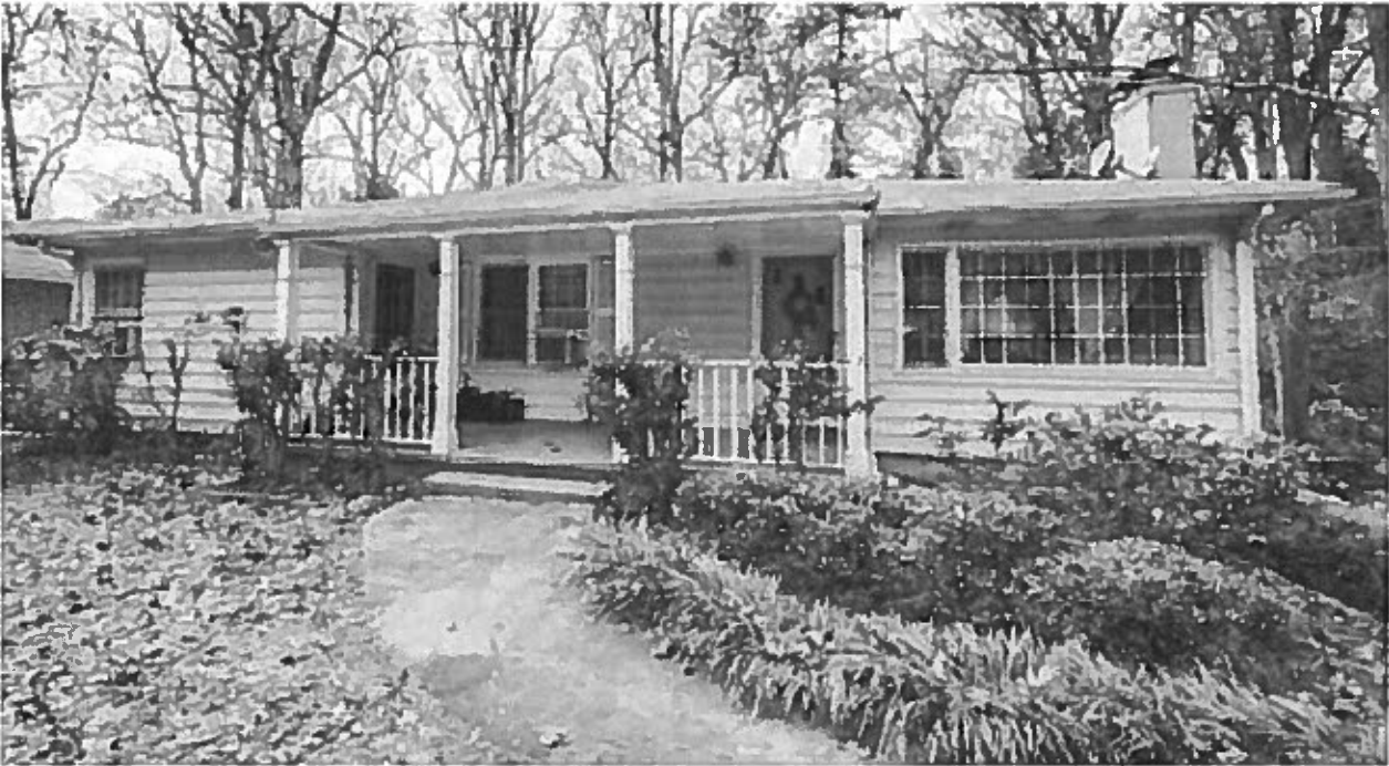
126 (128) Scott Blvd - elevations (photos)
