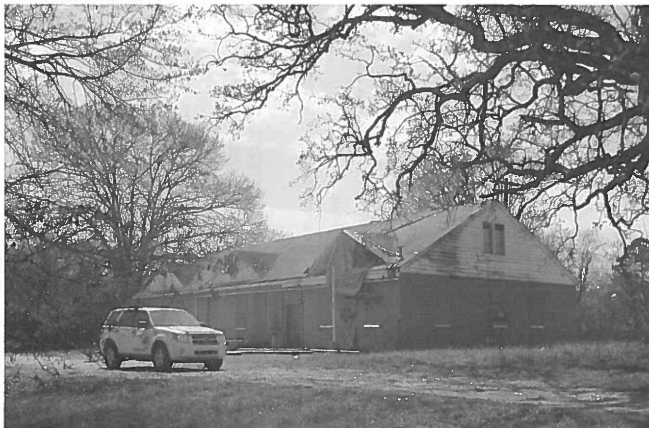
Front and north side of subject property.
