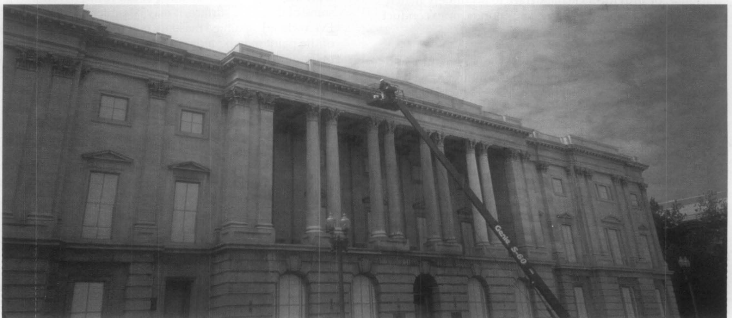
Figure 1. Low-to medium-pressure steam (hot-pressurized water washing), is being used to clean the exterior of the U.S. Tariff Commission Building, the first marble building constructed in Washington, D.C., in 1839. This method was selected by an architectural conservator as the "gentlest means possible" to clean the marble. Steam can soften heavy soiling deposits such as those on the cornice and column capitals, and facilitate easy removal. Note how these deposits have been removed from the right side of the cornice which has already been cleaned.
