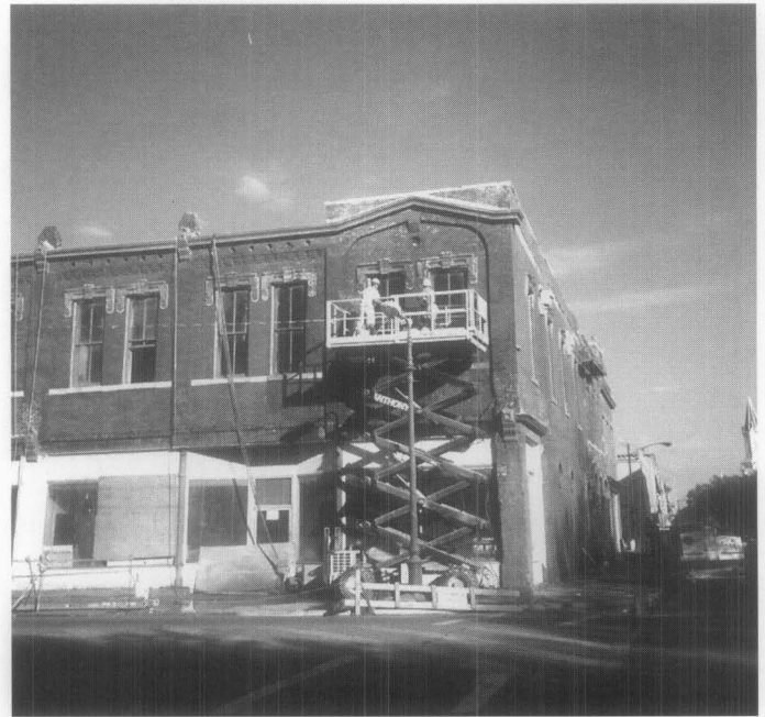
Figure 14. Chemical removal of paint from this brick building has revealed that the cornice and window hoods are metal rather than masonry.
