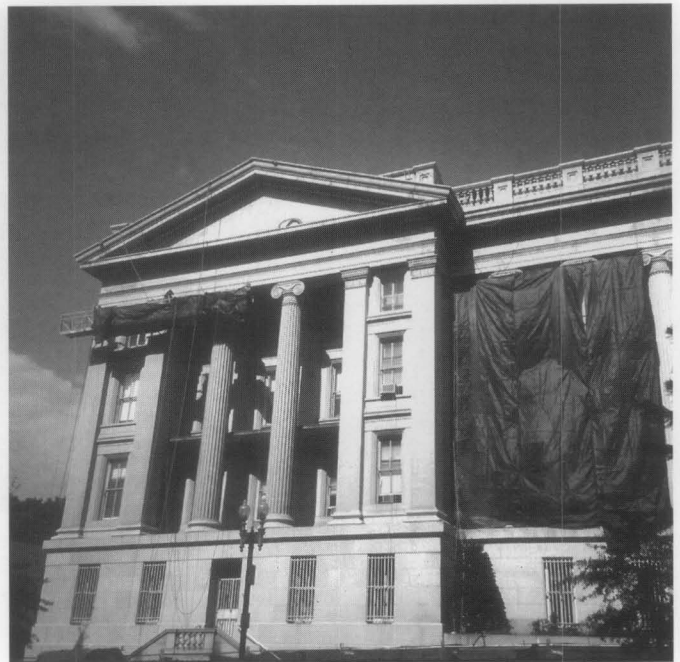
Figure 23. A tarpaulin protects and shields pedestrians from potentially harmful spray while chemical cleaning is underway on the granite exterior of the U.S. Treasury Building, Washington, D.C.
