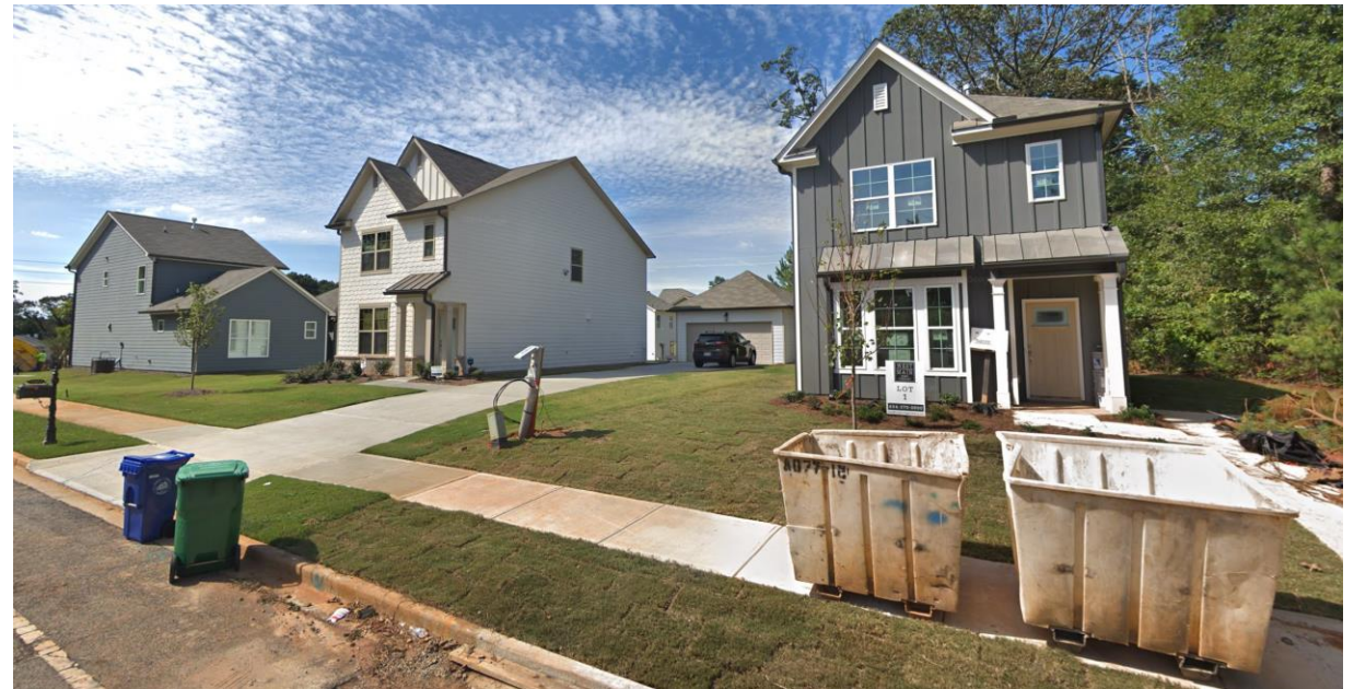
(right) Homes on nearby Windy Hill Road lots located to the south of the subject property.
