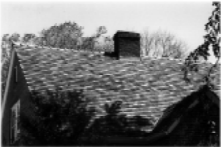
This interior brick chimney is a small but important element of the roofline of this house.
