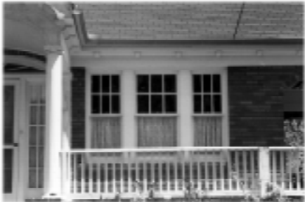
These double-hung windows, with six-over-one pane configuration typical of the Craftsman style, have been well-maintained.
