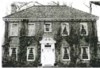
Good example of clay tile roof on Oakdale Road.
