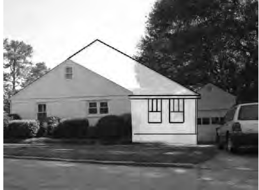
Poorly conceived addition that would mask the homes original proportions and character.
