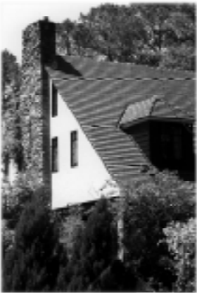
The random-stone masonry of this chimney is unusual in Druid Hills and should be properly maintained.
