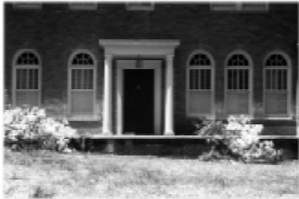
This group of round arched windows is a characteristic feature of the Italian Renaissance Revival style.
