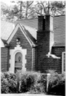
This front-facade brick chimney adds to the picturesque character of this English Vernacular Revival style house and should be maintained.
