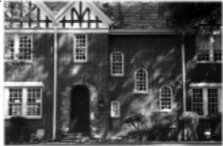
The row of stepped windows on this house provides the front facade with a distinctive pattern that should be maintained.
