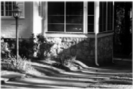
This granite foundation is characteristic of houses found in Emory Grove and should be properly maintained
