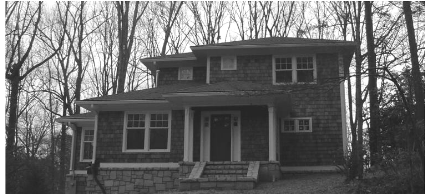
Well executed new construction (2008) in Chelsea Heights subdivision. Horizontal emphasis is maintained by judicious use of a hipped roof. Foundation is low (because of well conceived contour grading) and granite. Multiple architectural elements and roof setbacks avoid a monumental façade. Architectural details are important but minimal.
