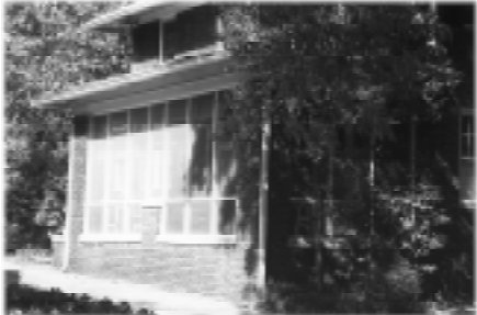
This side porch has been enclosed with screen, helping to maintain its original open character.
