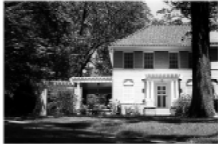
The open pergola design of this entrance porch, side porch, and porte cochere is a significant stylistic feature of this house and should be maintained.
