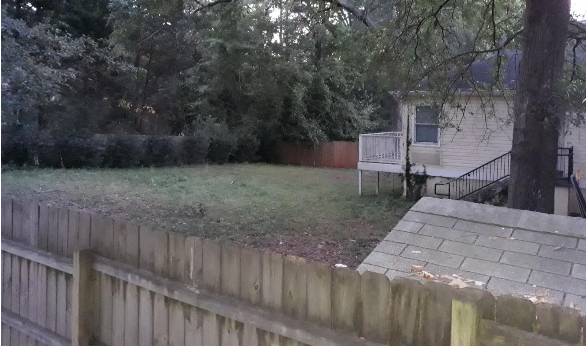
Rear of building and rear yard.
