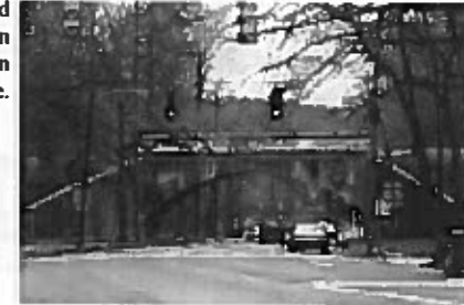
Railroad underpass on Ponce de Leon Avenue.
