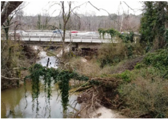
Existing conditions underneath the Orion Drive bridge facing South.
