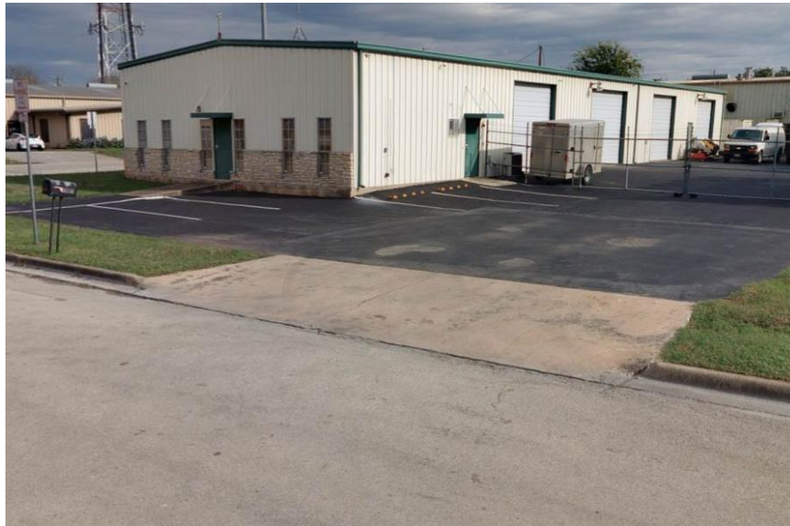
Figure 20: Example primary representative image of Warehouse and Loading Dock area
