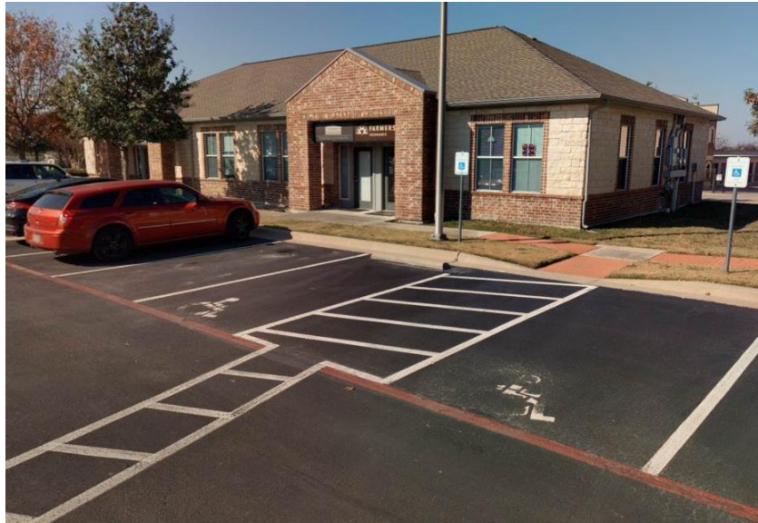
Figure 18: Example primary representative image of Building Type 1
