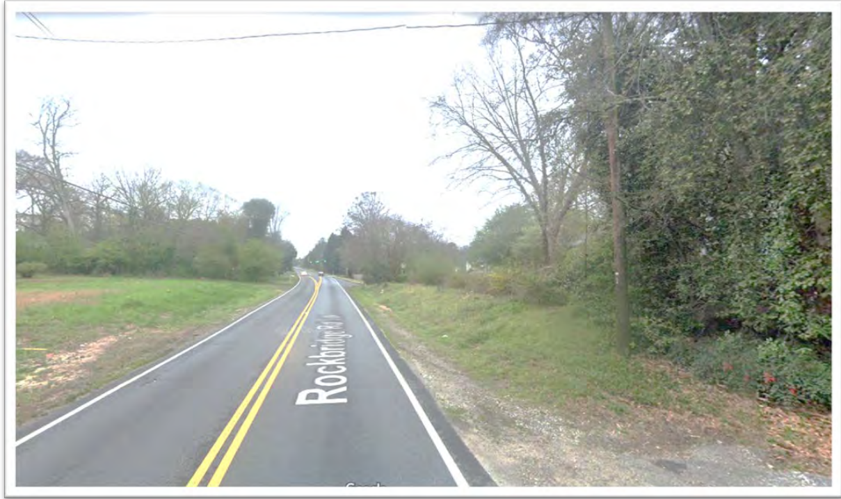
Photo 5 - Street Conditions Signalized Rockbridge Rd and Pennybrook Ln BirdsEye
