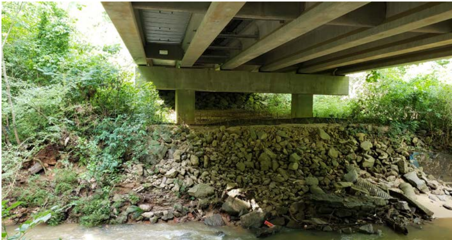
Existing conditions under Flowers Road, facing north. 8'-0" clearance for multi-use trail is achievable under Flowers Road
