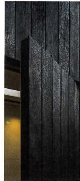
4: ROOF TERRACE WALL
