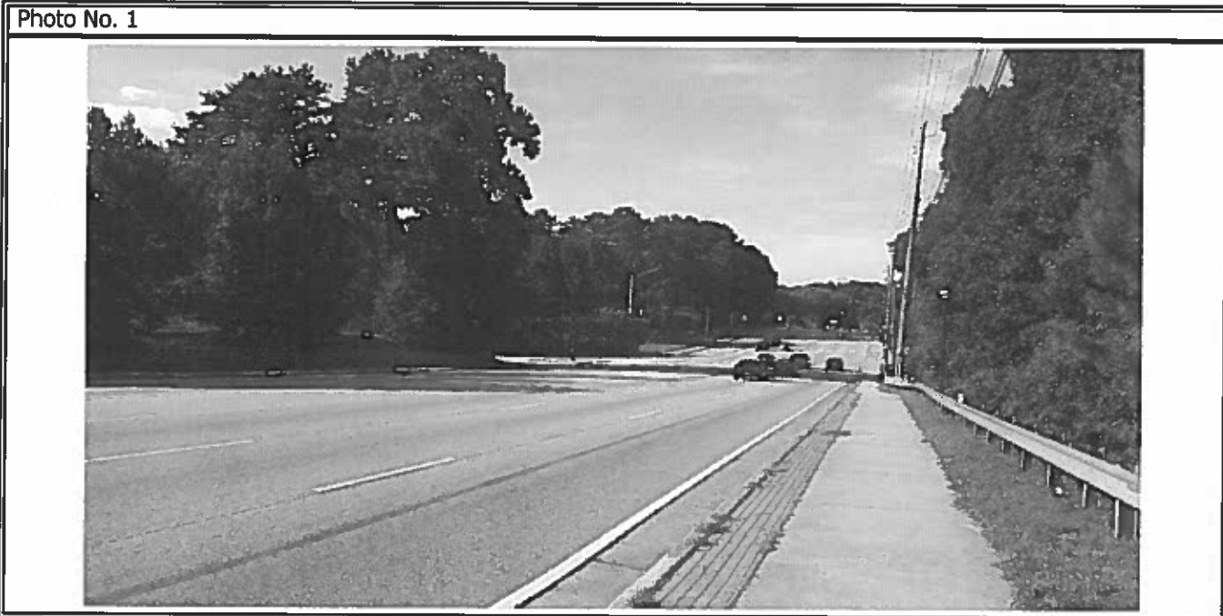
Comments: Site Driveway: Looking north along Memorial Drive (SR 154 / SR 10)
