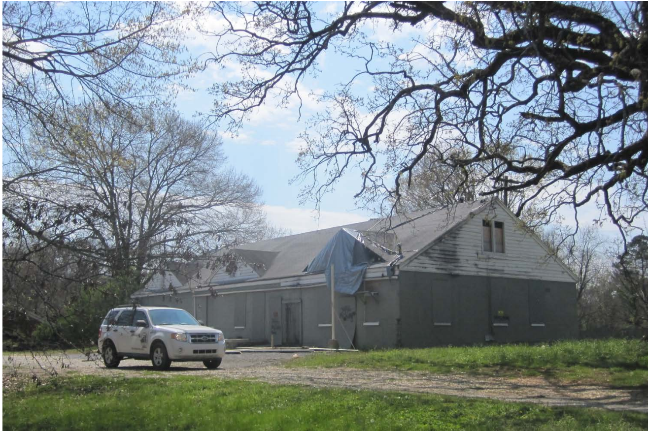
Front and north side of subject property.
