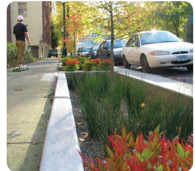
This cistern (above left) collects rainwater and stores for irrigation. The planting strip along this street is a 'rain garden' (above right) that filters stormwater runoff and recharges the water table, reducing the treatment costs for the City.
