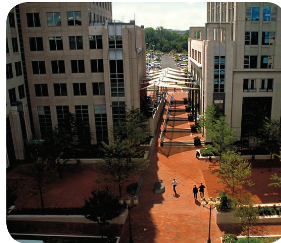
Deliberate massing ensures that the scale of an office building does not become overwhelming.
