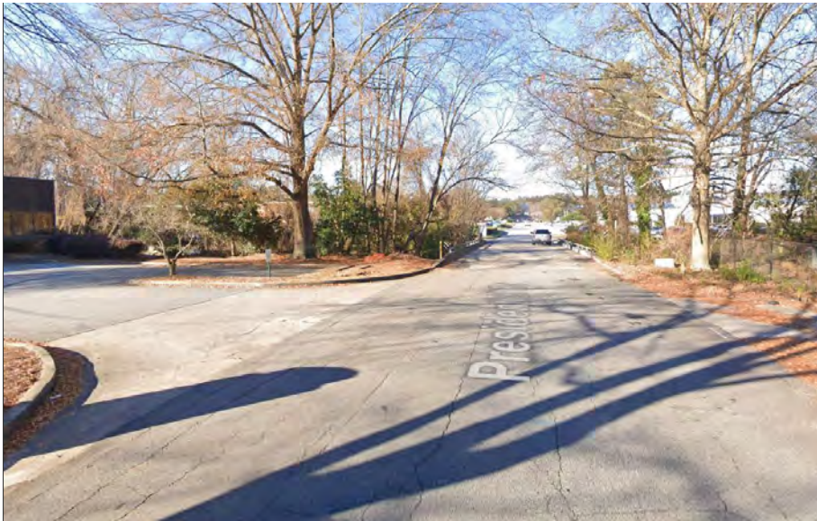
Existing conditions of Presidential Drive, facing west. A proposed at-grade crossing will connect the trail to the future redevelopment of the Clyde Industries parcels.
