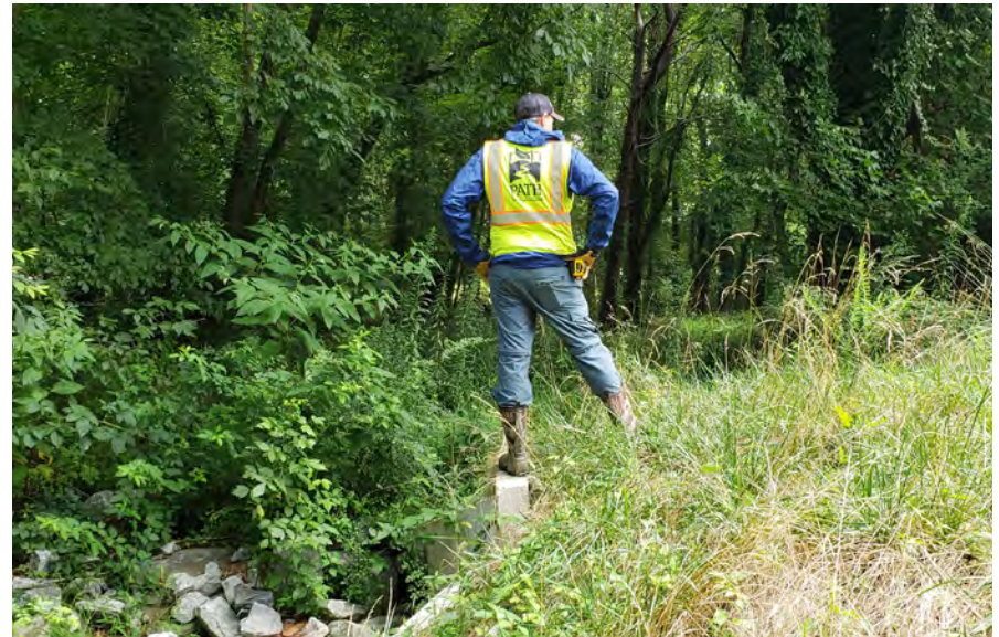
Existing drainage structure along sewer easement to the north of Century Center
