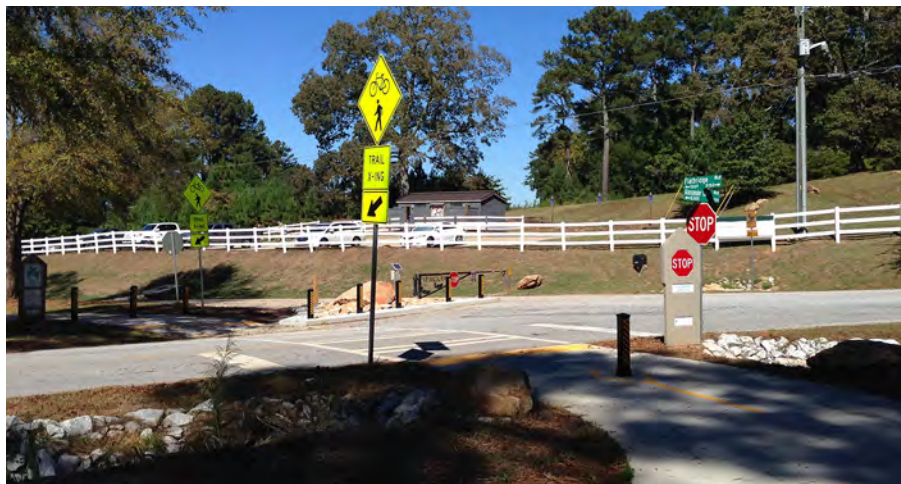
Typical trail intersection with signage, bollards, and pavement striping.
