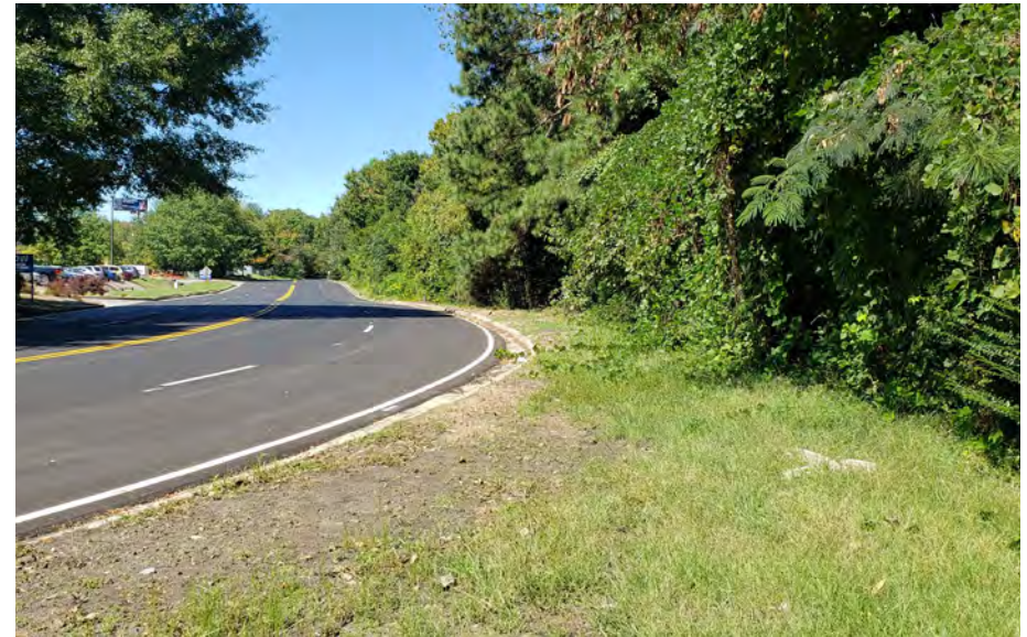
Existing conditions of Presidential Parkway, facing north-west. The proposed trail will meander through the greenspace between existing concrete and the creek as it approaches I-285.
