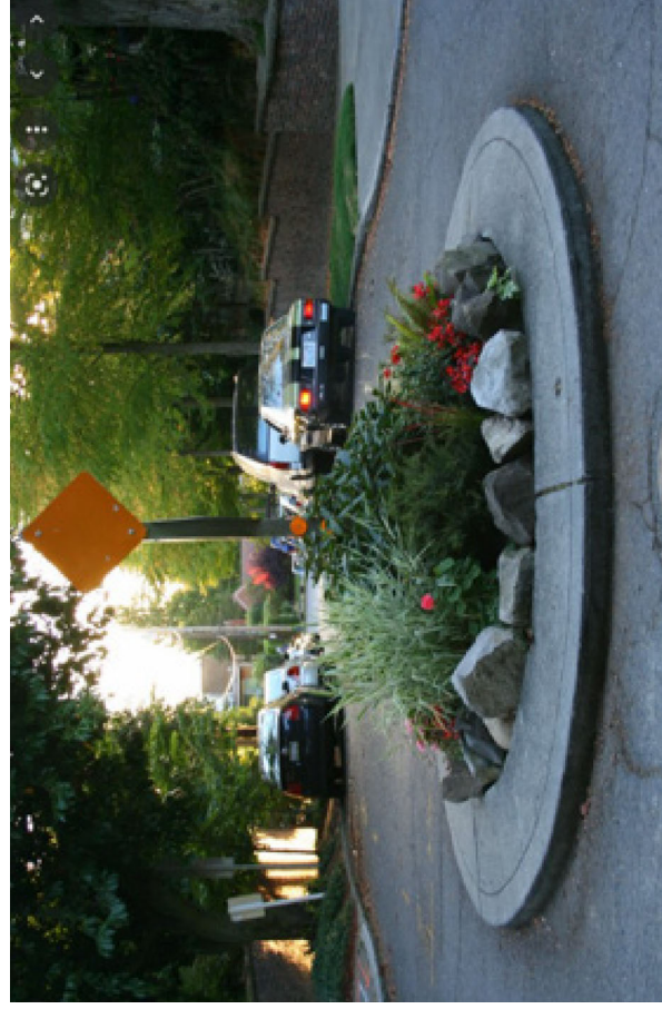
Calm Street example showing a Mini Roundabout as a traffic calming elements.
