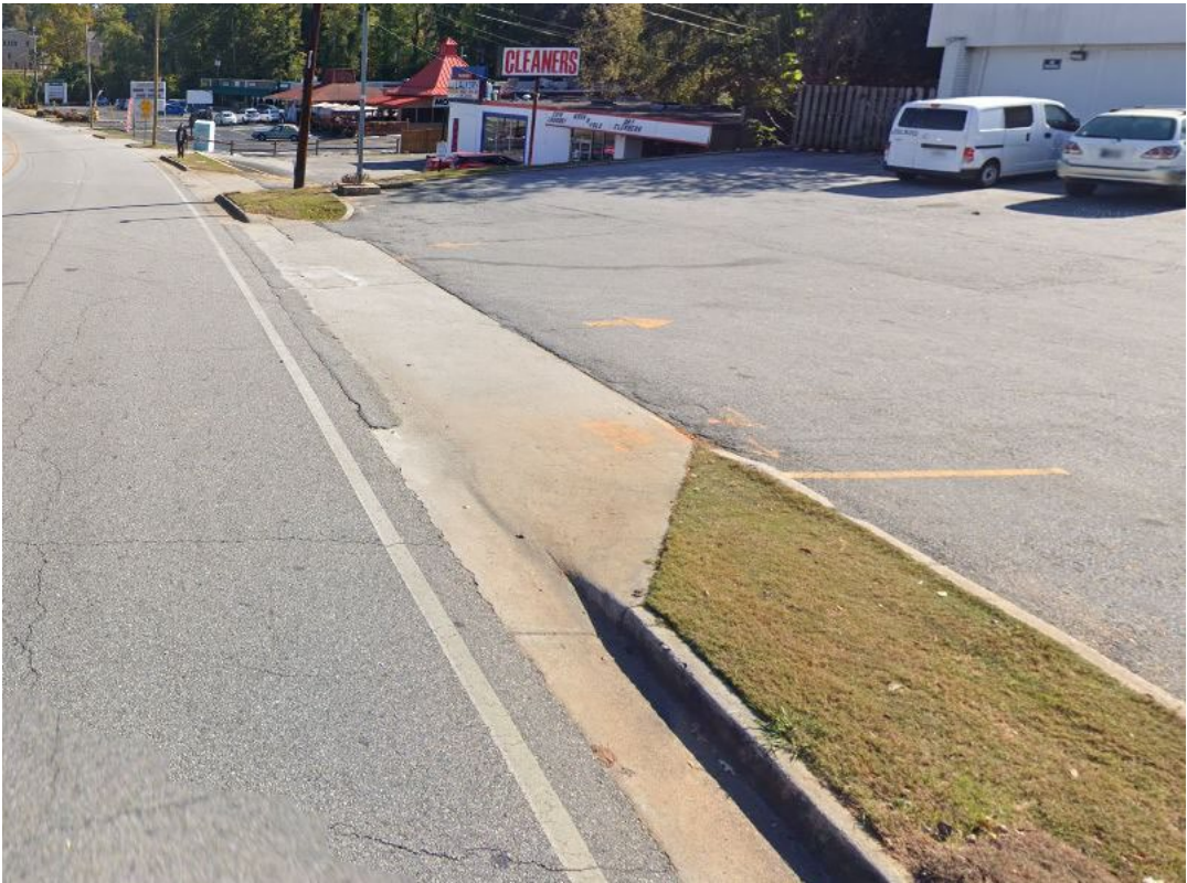
Streetscape and lack of sidewalk looking East on Briarcliff Road
