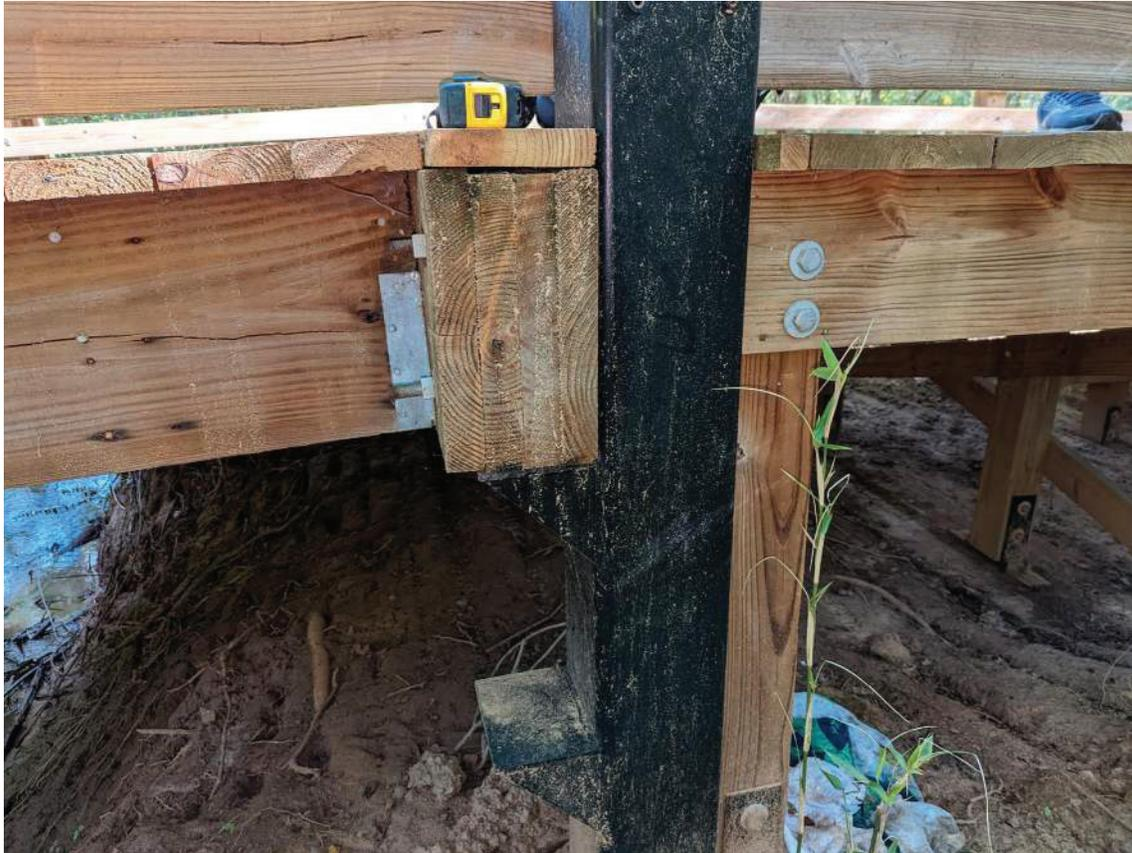
**Photo 4 – Bridge #1 Quadruple End Beam & Steel Post Connection**
