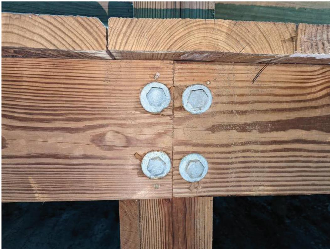
**Photo 8 – Boardwalk Post to Beam Connection (Typical)**
