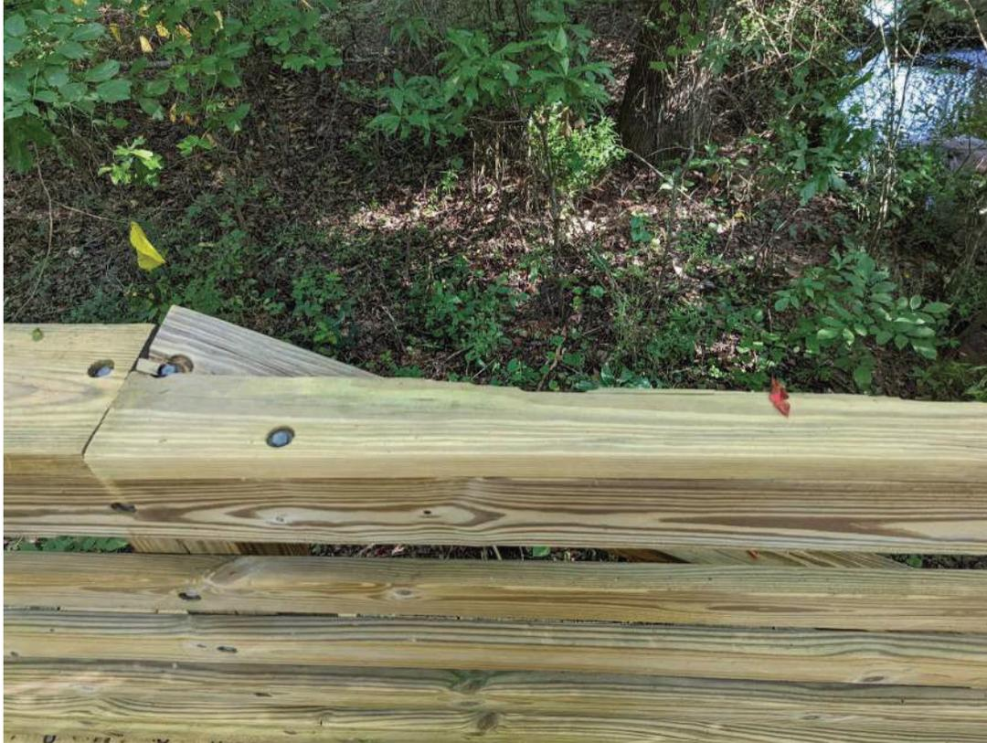
**Photo 9 – Boardwalk Handrail Cap Broken (Split Lengthwise)**
