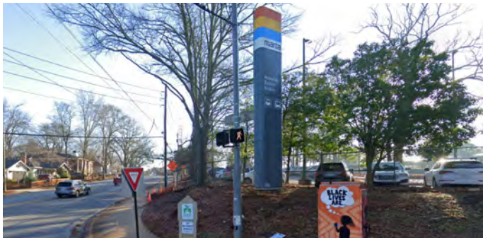
The Stone Mountain PATH crosses I-285 (top) and also connects to the Avondale Transit Station near Decatur (bottom)
