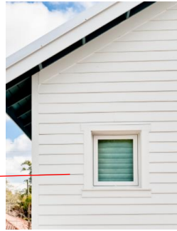
WHITE FIBER CEMENT BOARD SIDING LAPPED PATTERN
