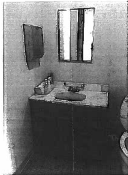
Office - Restroom Main Office - Bay 2 (First Floor)
