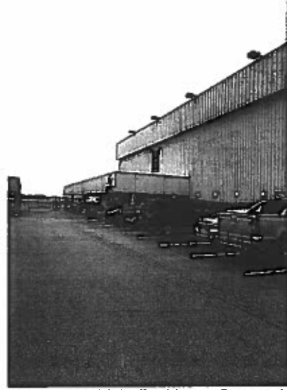
Asphalt Vehicle Parking – Covered Signature Flight Support
