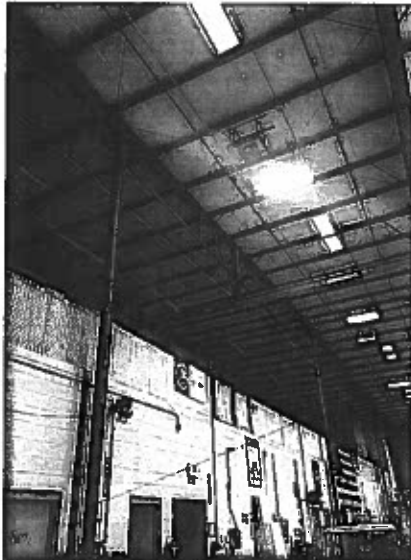
Shop and Storage – Interior Southern Company Hangar
