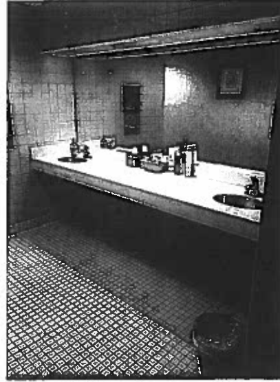
Office – Restrooms Southern Company Hangar
