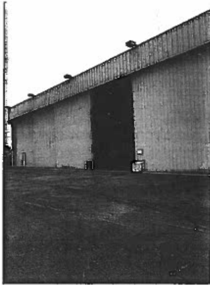
Hangar – Exterior Waffle House Hangar
