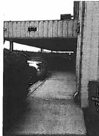
Asphalt Vehicle Parking – Covered Signature Flight Support
