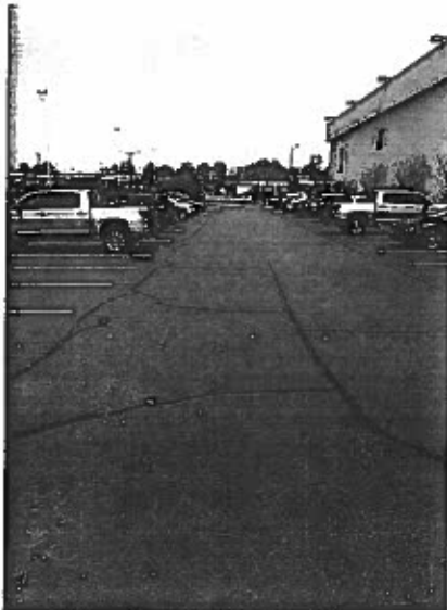
Asphalt Vehicle Parking Southern Company Hangar
