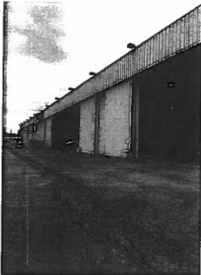
Hangar – Exterior Main Hangar – Bay 1 and Bay 2
