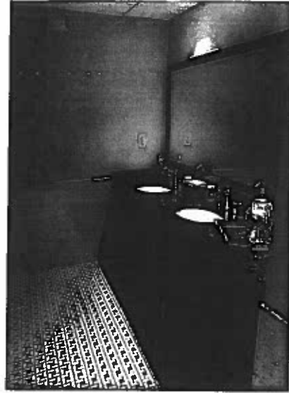
Office – Restrooms Main Hangar – Bay 1
