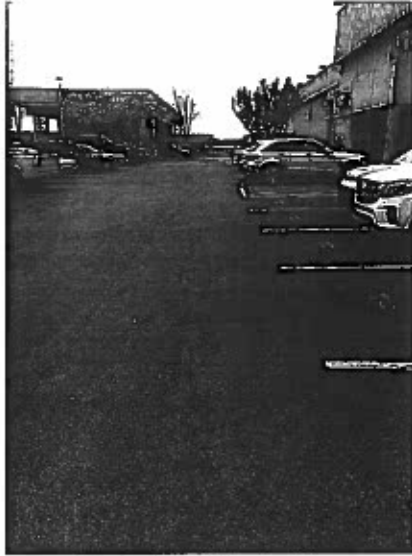
Asphalt Vehicle Parking Signature Flight Support
