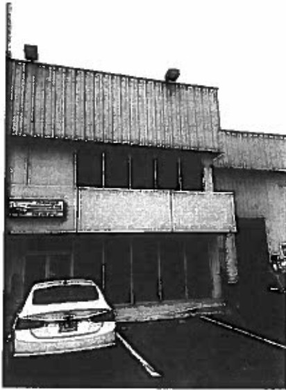
Office – Exterior Main Office – Bay 2 (First and Second Floor)
