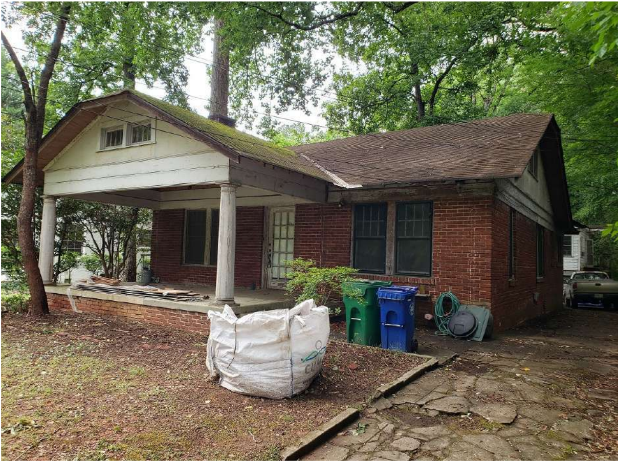
Front showing dilapidated driveway and non-historic columns and gable finish
