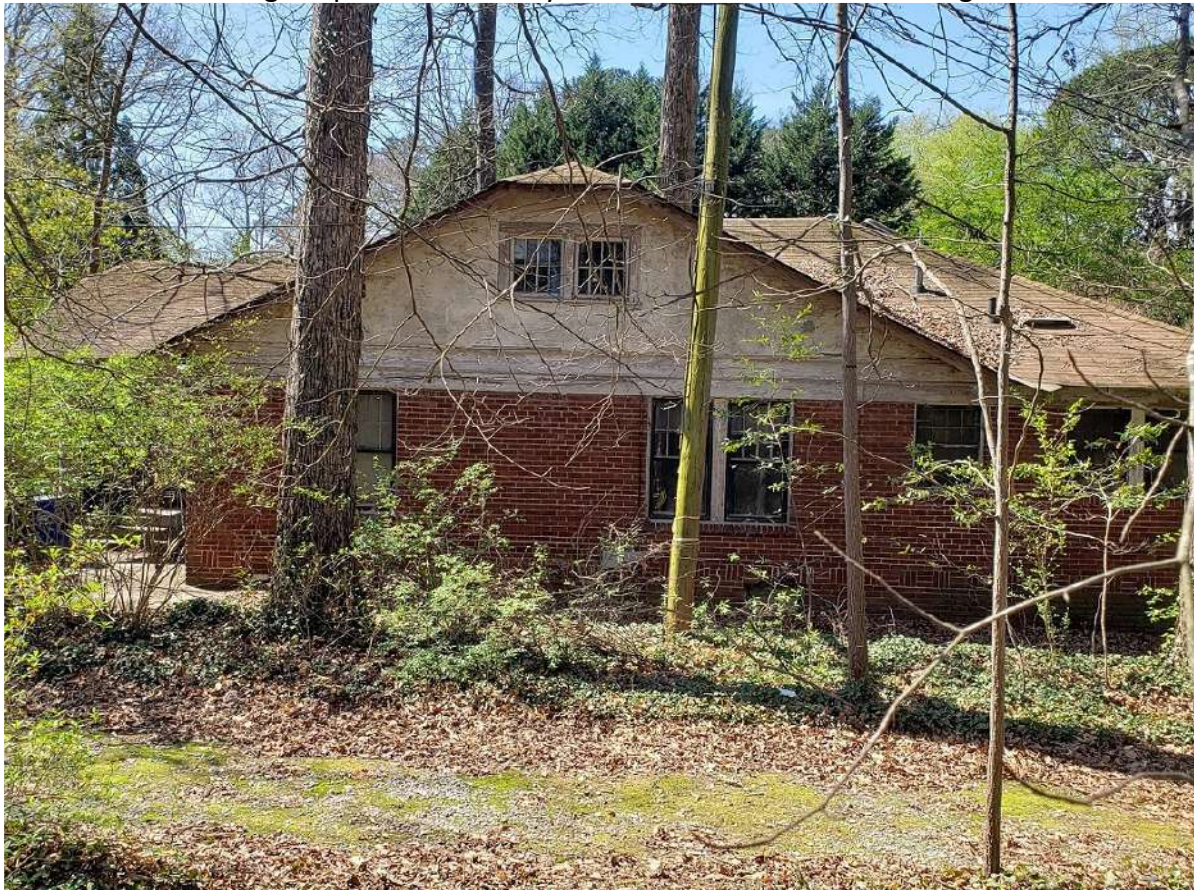
Right side and non-historic gable finish
