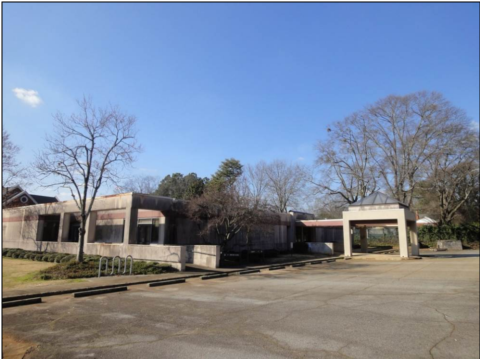
View of the subject property facing northwest from Church Street
