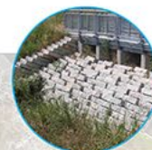
ENERGY DISSIPATOR TO PREVENT SOIL EROSION AND TREE LOSS
