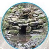
ENERGY DISSIPATOR TO PREVENT SOIL EROSION AND TREE LOSS
