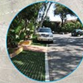
ON-STREET PARKING WITH PERMEABLE PAVERS TO INFILTRATE STORMWATER AND REDUCE EROSION
