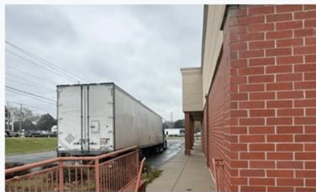
Photo 3: Deteriorating building facade
