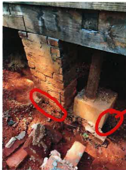
Figure 2 Brick pilaster isn't supported on concrete footing. Pipe post added to the right, but the footing isn't supported fully on soil.
