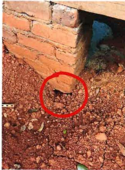
Figure 1 Void at bottom shows no footing
