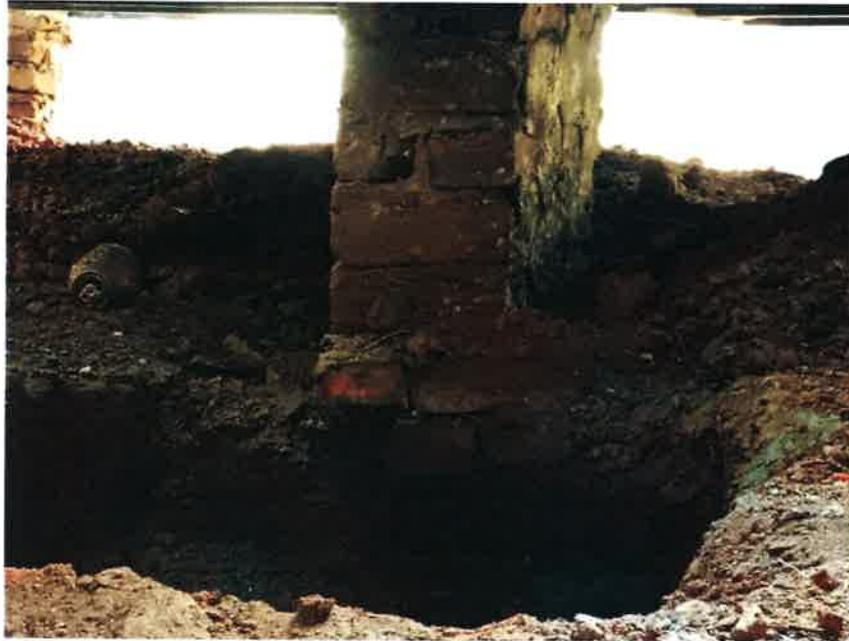
*Figure 3 Excavation shows no footing for brick pilaster*
