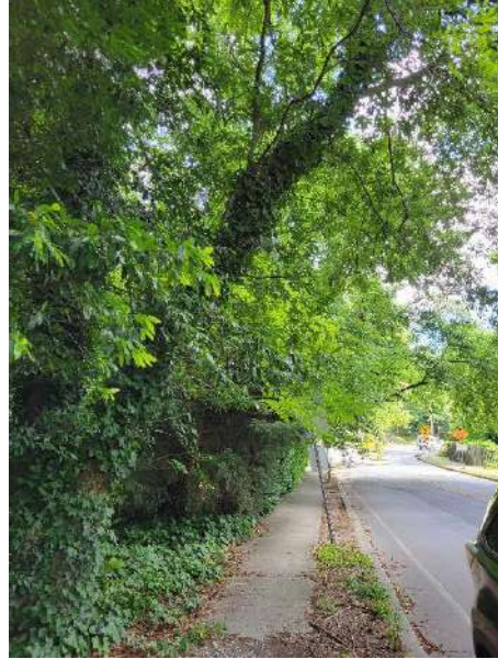
Tree 36 leaning over street
