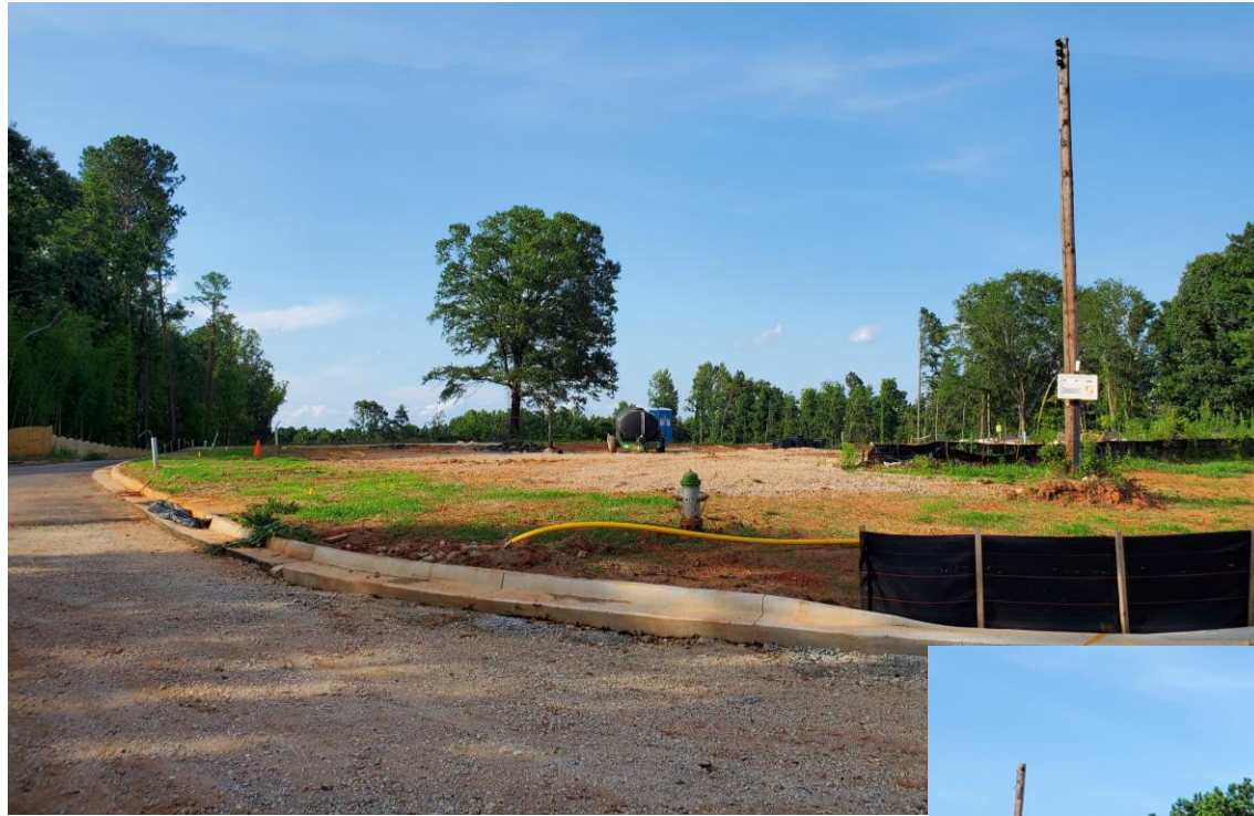
Front of subject property on Mountain Drive.
