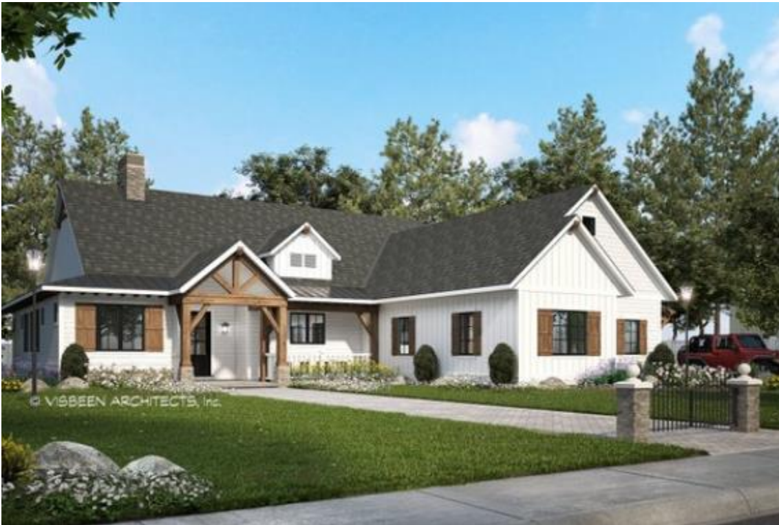
Trussed front porch
