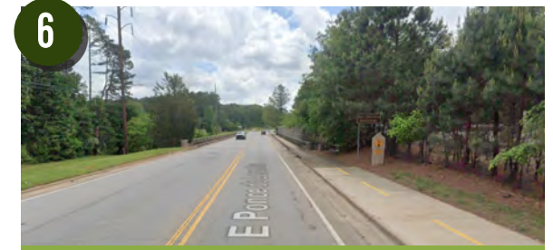
E Ponce de Leon Ave Bridge
