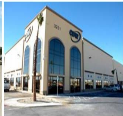
513,000-square-foot distribution center in NV
