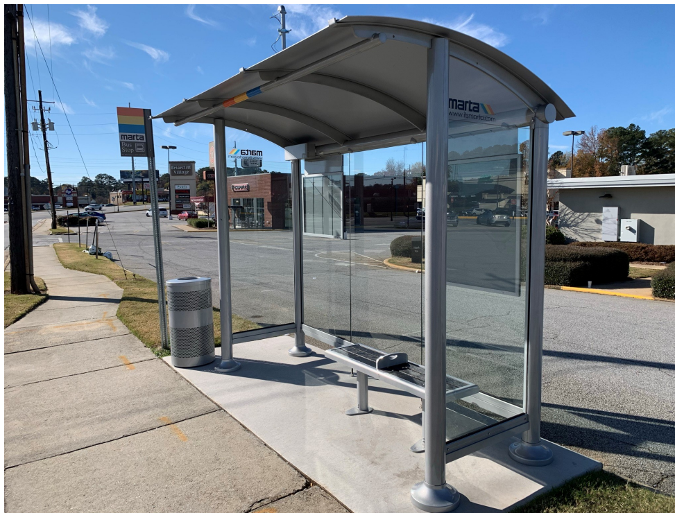
New MARTA Bus Shelter on Henderson Mill Road
