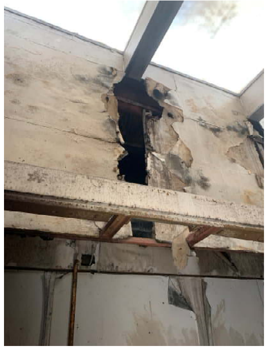
Skylight Area (MM-3 and MM-4)
