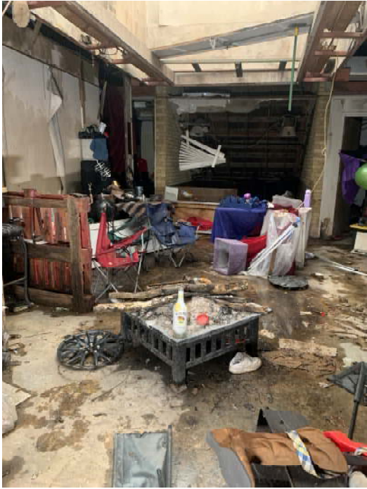
Skylight Area (MM-3 and MM-4)
