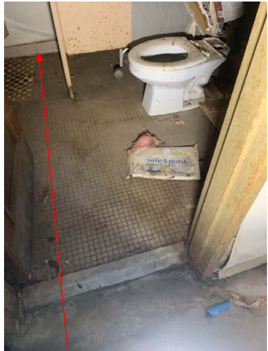
Bathroom #3 (MM-21), same tile present in Bathroom #1 and Bathroom #2
