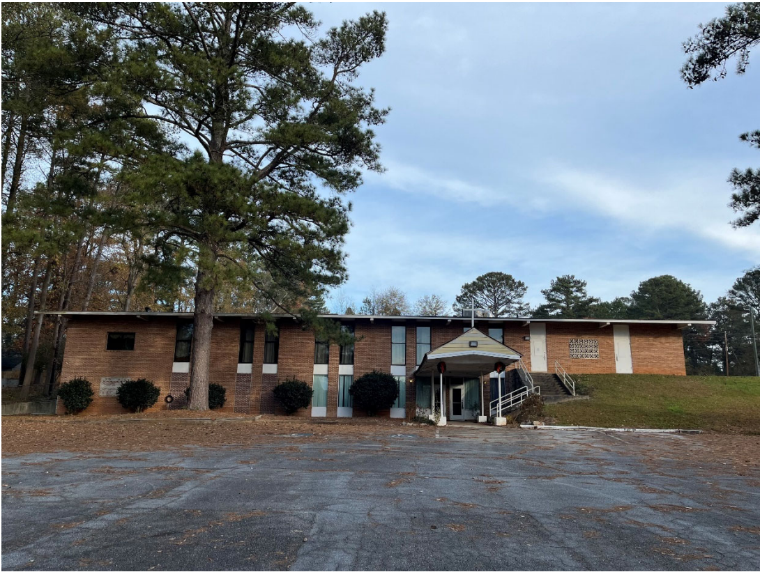
Existing south elevation as seen from the parking lot:
