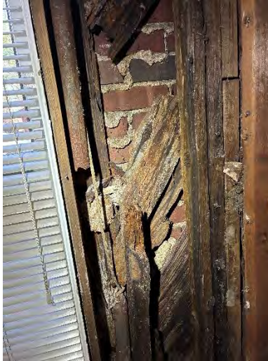
Photo 44 Northwest Corner Framing At Sunroom / Enclosed Porch
