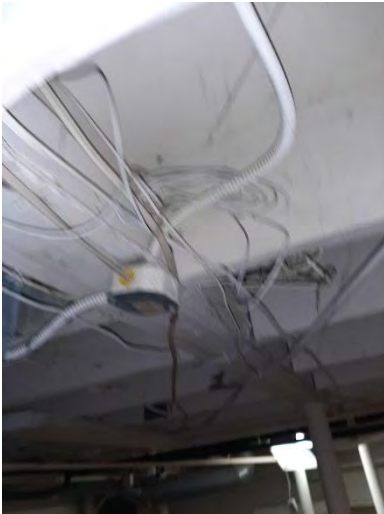
Photo 25 First Floor Framing
