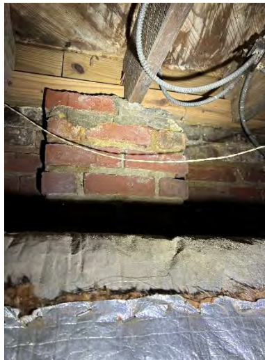
Photo 34 Brick Pilaster at Crawlspace
