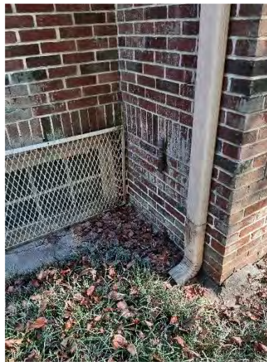
Downspout Near Basement Window
