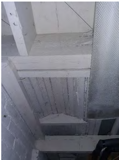
Framing Under Hearth
