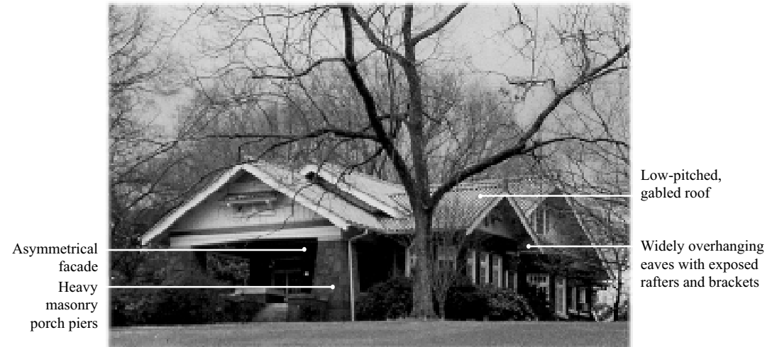
Excellent example of the Craftsman style with principal features keyed.
