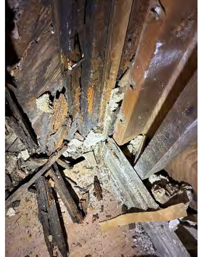
Photo 45 Northwest Corner Framing At Sunroom / Enclosed Porch
