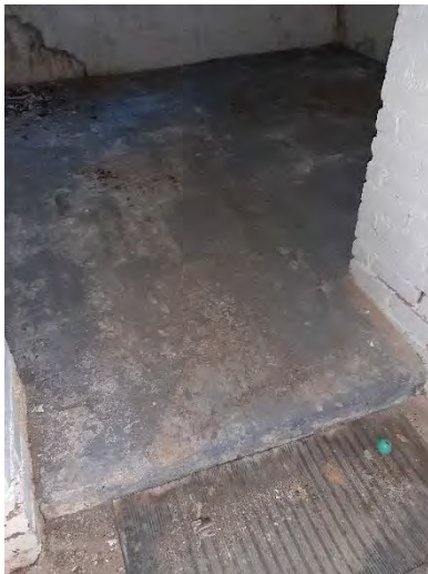
Photo 36 Slab on Grade
