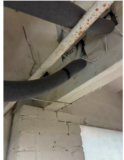
Photo 27 Header Beam at Stair Opening
