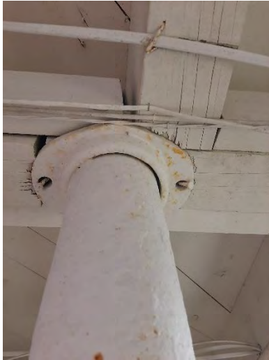
Photo 28 Top of Pipe Column
