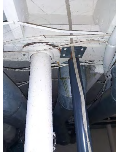
Photo 30 Top of Pipe Column With Adjacent Shoring Post
