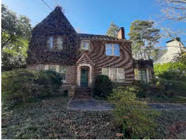
Photo 1 Front of House (East Façade)
