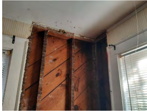
Photo 17 Second Floor Wall
