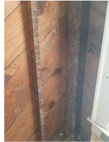
Photo 18 Second Floor Wall
