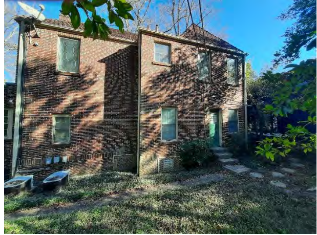
Photo 2 Rear of House (West Façade)
