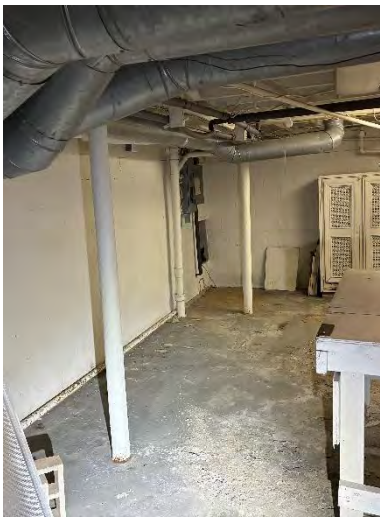
Photo 37 Slab on Grade
