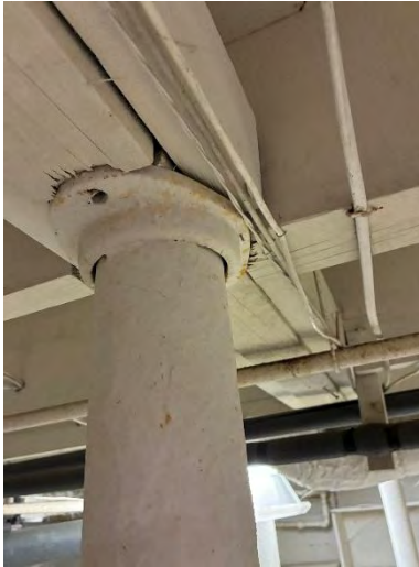
Photo 29 Top of Pipe Column
