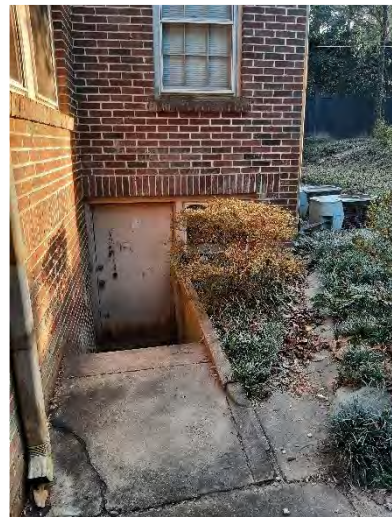
Photo 38 Exterior Basement Entrance
