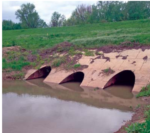
The aging and failing levee before SAK Construction's SPR solution is installed.
