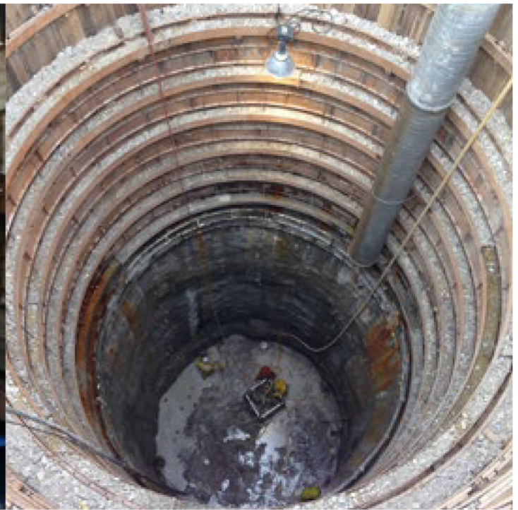
Shaft Excavation
