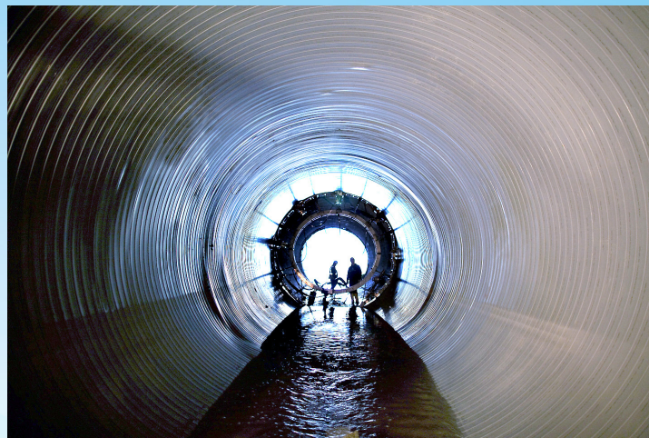
Spiral Wound (SPR) after rehabilitation
