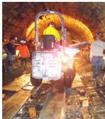
SAK Construction LLC, recently began work on rehabilitating a 5,575-lf segment of the Old Mill Creek Sewer in Downtown St. Louis.
