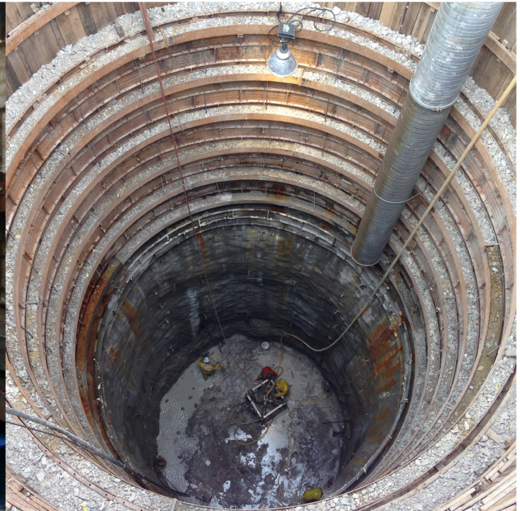
Shaft Excavation
