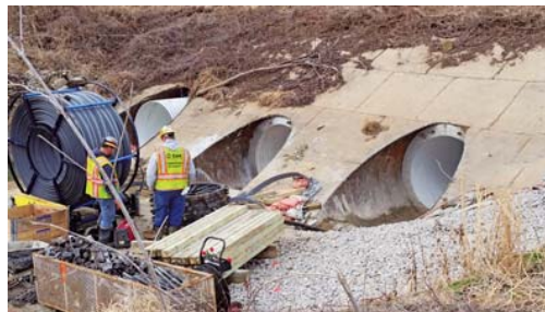
SAK started installing SPR in the upstream sections of the pipe and during the winding process diverted the flow among the three 84-in. corrugated metal drainage pipe sections until each 150-lf section was wound, bulkheads and bracing installed, and structural grouting commenced.
