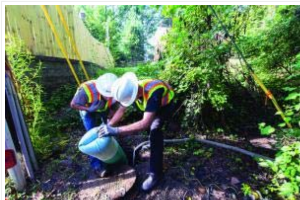
Kyle Bowen (left) and Zach Andrews of SAK Construction guide the terminal end of a CIPP liner out of a manhole on a sewer relining job in St. Louis.
