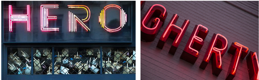
OPTION 7A: Exposed Neon Mounted Directly to Façade OPTION 7B: Exposed Neon Mounted on Solid Letter Forms
